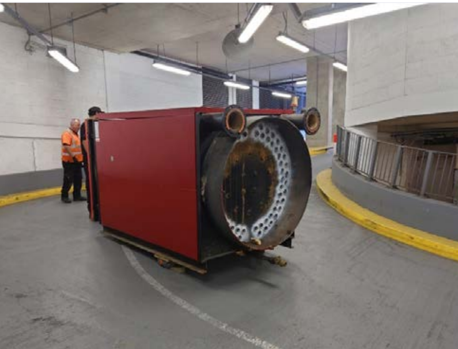
Boiler removal
