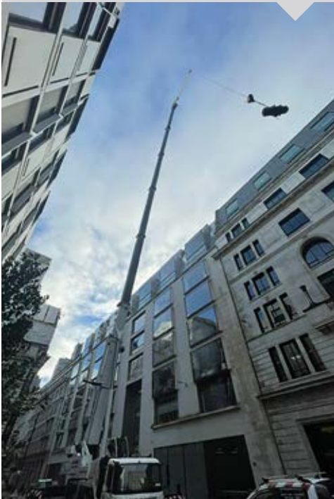
The crane lift was a great team effort
