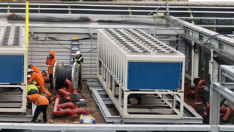
A new steel frame is being installed
